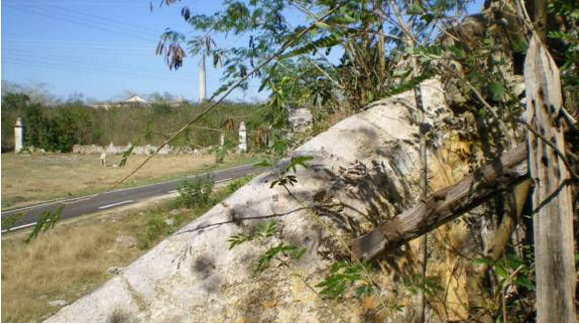
The view from the mansion steps of the massive henequen processing plant is nearly swallowed by the encroaching jungle and only the roof and smokestack can be seen.
